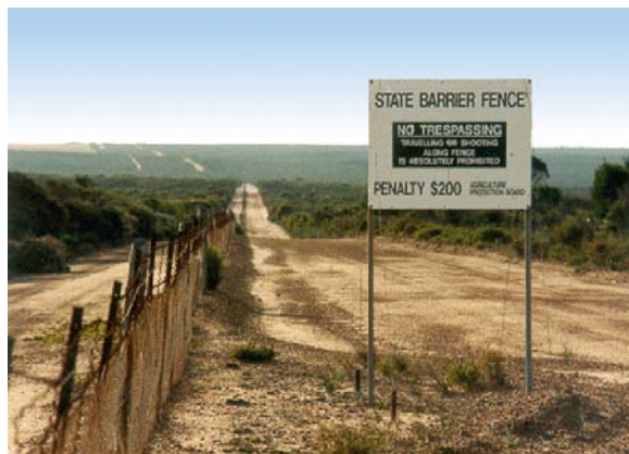
Figure 3 The “Rabbit Fence” 100 years after construction.
