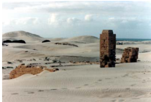
Figure 2. Drifting sand at Eucla now covers the formerly high walls of the overland telegraph station to the extent that only the chimneys protrude.
